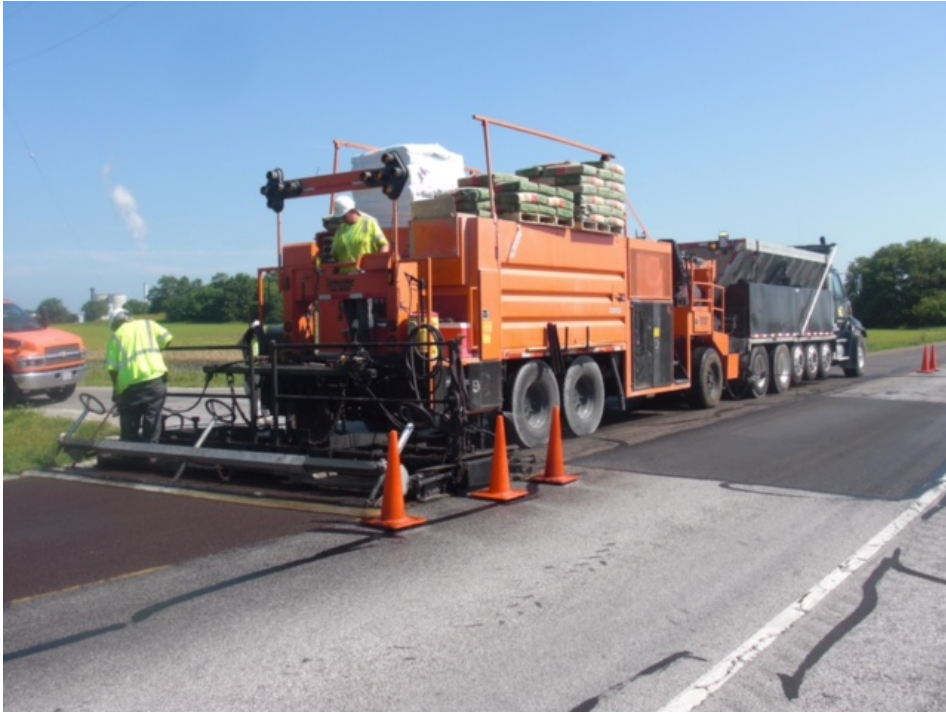
Microsurfacing paver in operation.
