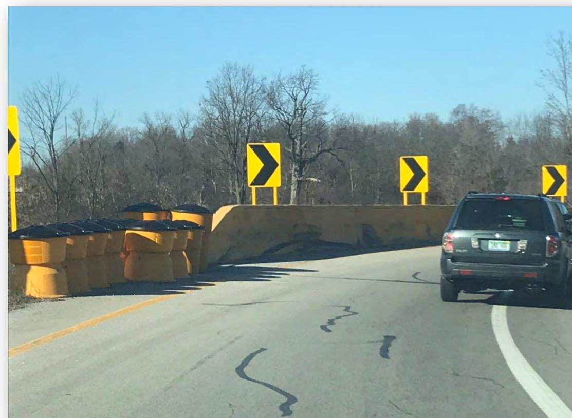
Although a safety issue is not evident on the interchange ramps based upon the crashes obtained from ODOT's GCAT tool, the strike marks observed on the northbound off ramp barrier are concerning. Modifications to the ramps should be considered because any improvements to the ramps provided by the proposed interchange alternatives could improve safety at the adjacent intersections as well.
