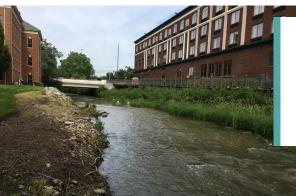
Urban stream channels can sometimes become overwide. When this happens, the flowing water contributes excessive stress on streambanks, causing them to be undercut and slough into the stream.
