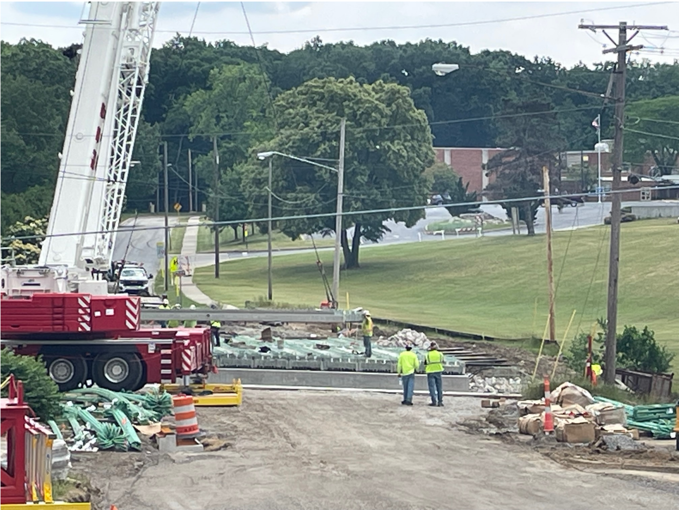
Silica Bridge Construction – June 13, 2023
