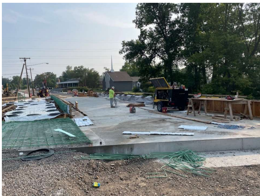
Silica Drive Bridge Construction
