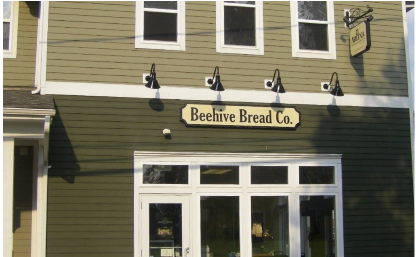
➡ Exterior lighting accents the building and makes the sign easier to read at night.
